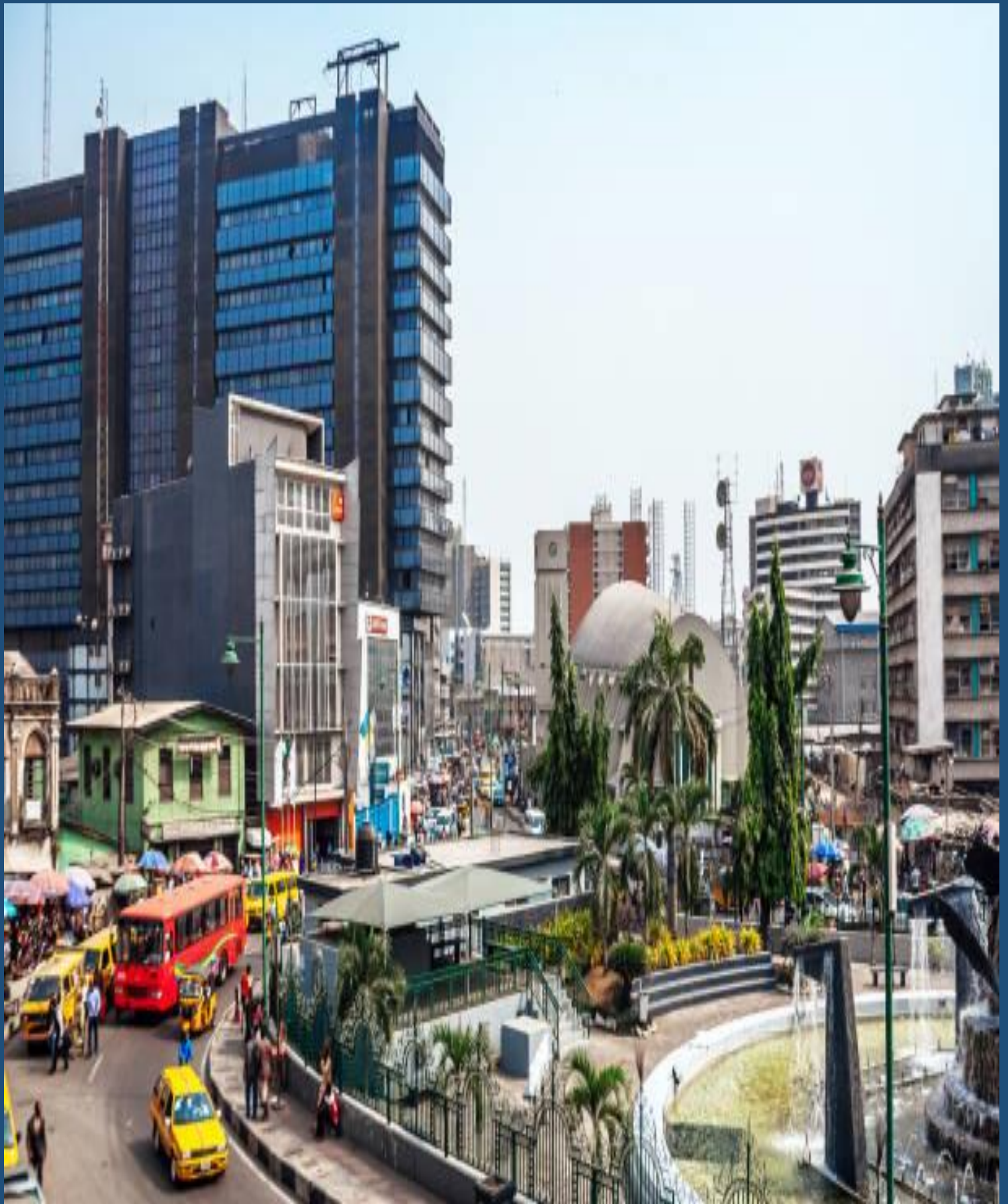
Lagos, Nigeria: Tinubu Square on Lagos Island - surrounded by high-rise buildings, park and fountain in the middle Image source: Istock
